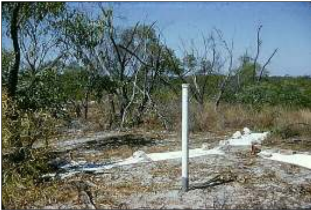
'Witness post adjacent to panelled control station'
