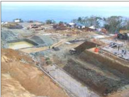
*The project started mid July with 90% of the access roads & earthworks for the process plant area now complete. The construction of the process plant is well under way with mining due to start in January 2005 and the first gold pour schedule for April/May 2005.*
