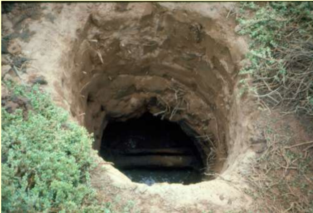
Midway Well - with timbers and water starting to fill the well
