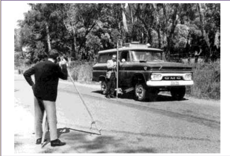
Levelling to get elevation of 'fifth' wheel
